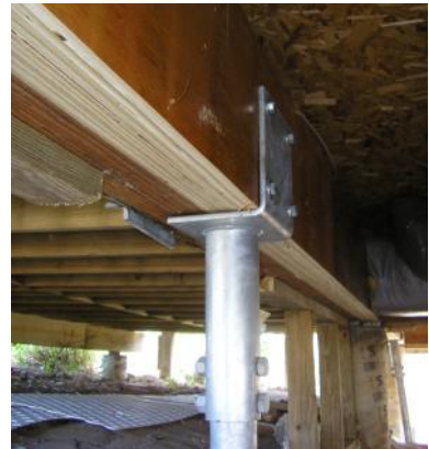
The photographs above show the pile installations being completed in the tight conditions under the structure.
